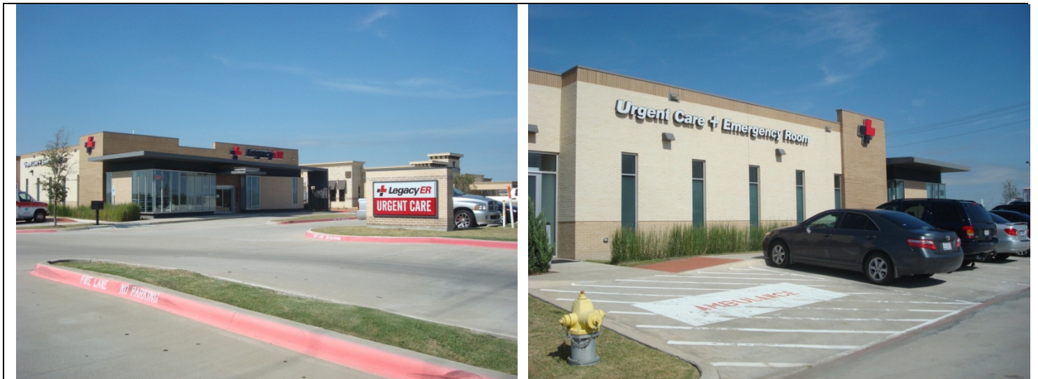
Figure 5.0: Legacy ER and Urgent Care Center, Frisco, Texas
